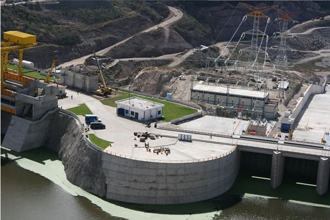
Honduras' state power company ENEE begins discharges at hydroelectric dam El Cajón. (source: Bnamericas Nov 6, 2020)
